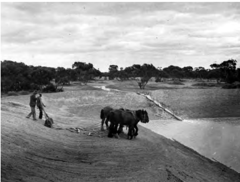
Creating water storage using horse scoop c.1940
