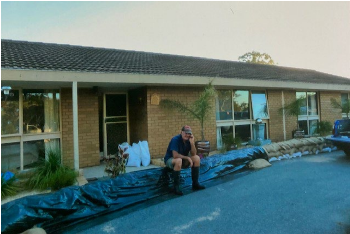
Photo 2 - 19/01/2011 126 - 128 Craig Ave Fully sand bagged. Flooding through drainage pipes.
