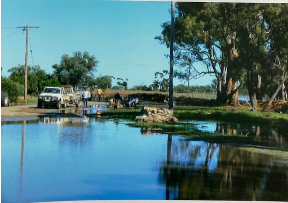
Photo 3 - 19/01/2011 128 to 132 Craig Ave, blocked entrance to Lots 4 & 5. Sandbags stopping town drainage from back flooding.
