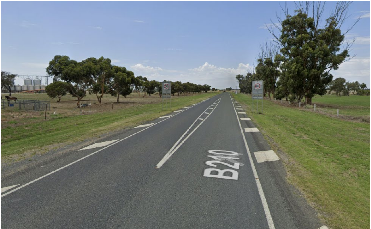
Figure 2: Southbound view of Stawell-Warracknabeal Road which adjoins the subject site, 21 Church Street Minyip.
