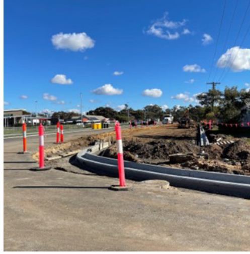
New kerbing in Werrigar St Warracknabeal
