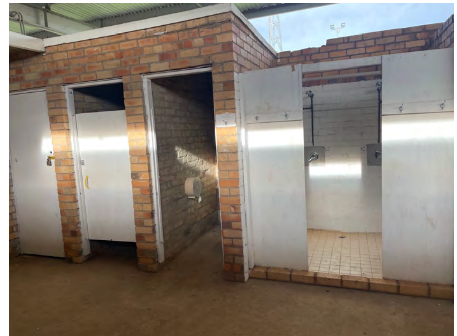
Figure 11: Men showers and cubicles. Warracknabeal Swimming Pool
