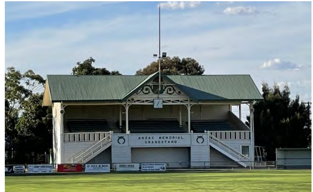
Figure 10: Grandstand at ANZAC Reserve oval
